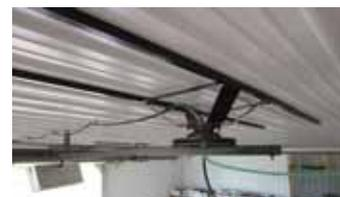
air hose and electric cord run down from ceiling through a pvc tube that runs through a car wheel axle bearing.
