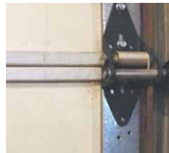
Spring-loaded garage door hinge pushes door gap shut to keep heat from leaking outside.
