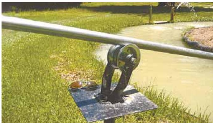
Pipe rides on a small metal roller mounted on a pedestal base.
