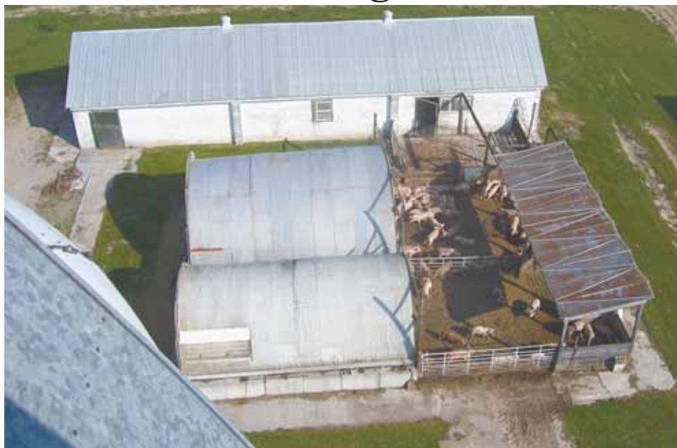
Eric Hartemink converted 2 old grain bins into inexpensive, "quonset-style" hog shelters. He tipped the bins on their side and removed the roofs, then mounted the roofs on metal posts to create a carport-like shelter that covers his feeders.
