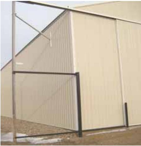
On windy days, the 20-ft. sq. doors on Gutschmidt's machine shed would catch wind like a big sail. The sliding door supports he designed keep that from happening.
