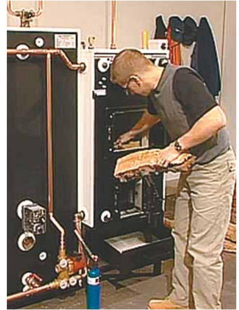
Imported “smokeless” wood boilers use the energy available in wood twice as effectively when compared to traditional wood boilers, say manufacturers.
