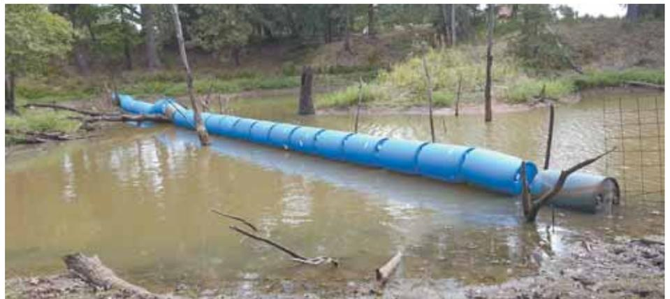
Barrel fence solves the problem of trash catching in wire and other types of fencing. The threaded-together barrels tend to roll right over it.
