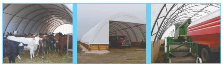
Steel series of hoop buildings is available in 30-ft. wide single hoops, and 30, 38, 42, 50 and 65-ft. wide truss arches.
