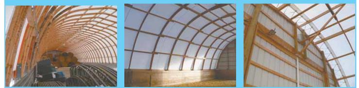
Silver Stream makes hoop barns with either steel or wood hoops. The advantage of wood is that it's easier to insulate and it can be tinned over at any time, if desired.
