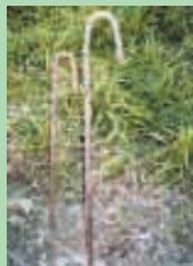
To hold the panels in place they bent lengths of rebar into the shape of “candy canes”.
