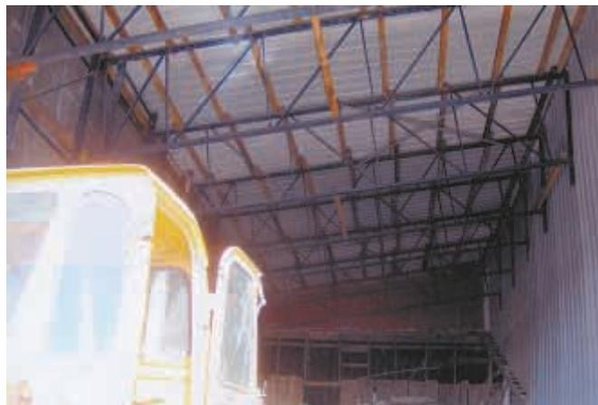
Used industrial shelving was used to form trusses and walls on Mark Musser's add-on building. The 5-ft. wide panels are 22 ft. long and are made from 4 by 3 channel iron.
