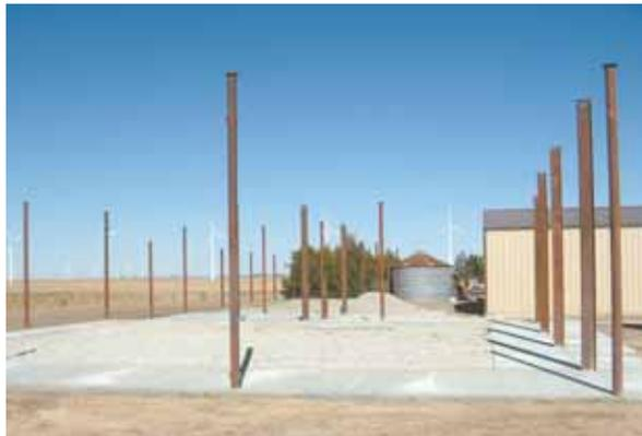
Doug Dumler used old center pivot pipe for the framing on his home-built, 60 by 60-ft. shed. Photo shows vertical pipes placed in cement-filled holes.
