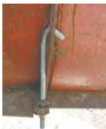
Turnbuckles attach to each end of pipe to hold it in place.
