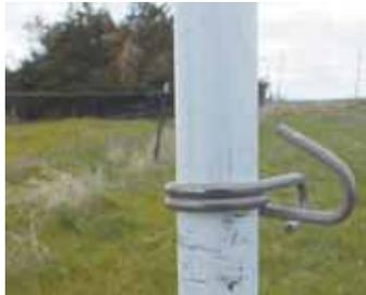
Electric wire is held on with a steel clip that slides over the post.
