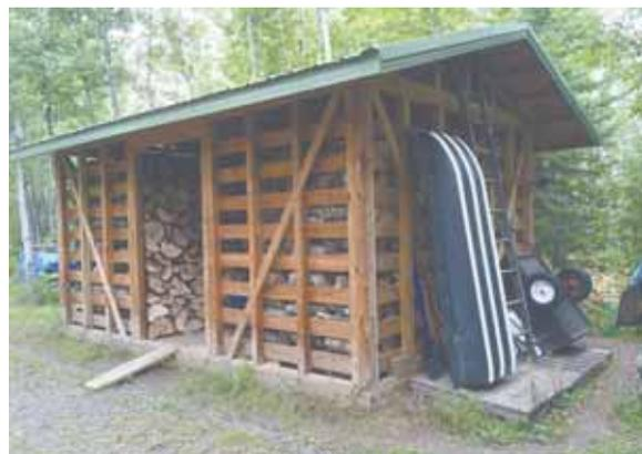
Heavy-built shed has 4 by 4 corner posts with 2 by 6 wallboards spaced 8 in. apart.
