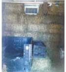
Air conditioner hangs from a hole cut into an outside wall of the shed, which is covered with bales on the inside. A CoolBot controller keeps the temperature low.
