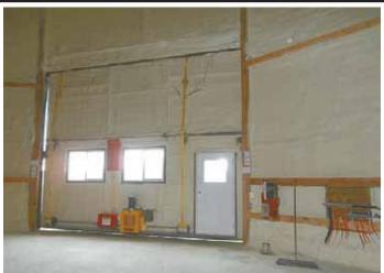
Measuring 16 ft. high and 20 ft. wide, bifold door is complete with windows and a walk
