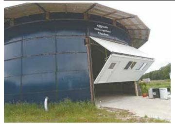
Marv Rubingh converted his 23-ft. tall, 62-ft. dia. Slurrystore into a shop complete with a Schweiss bifold door and barn steel roof.
