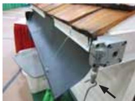
Hooked handle turns gearbox at one end to bring gutter up to catch rain and let it down to drop leaves.
