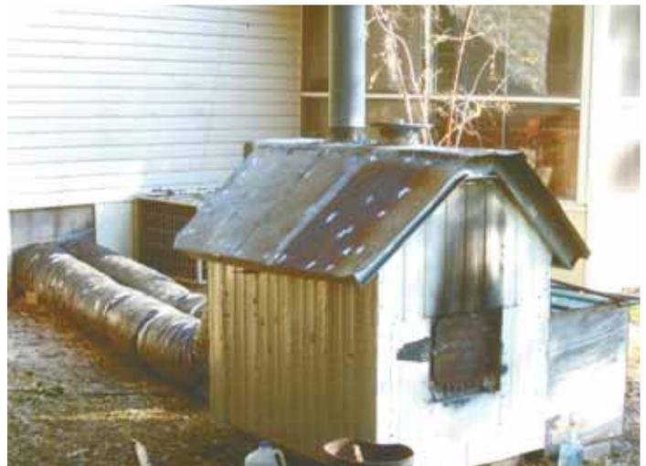
Barrel stove is surrounded by an aluminum housing that gathers heat off the stove. Insulated flexible heat ducts carry the heat inside Dreifus’s house.
