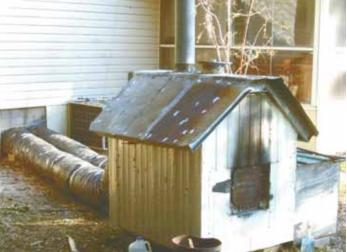
Barrel stove is surrounded by an aluminum housing that gathers heat off the stove. Insulated flexible heat ducts carry the heat inside Dreifus's house.
