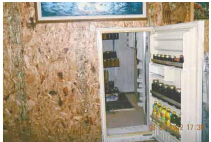
Refrigerator door mounted in cellar wall was a low-cost way to provide an air-tight entrance point.
