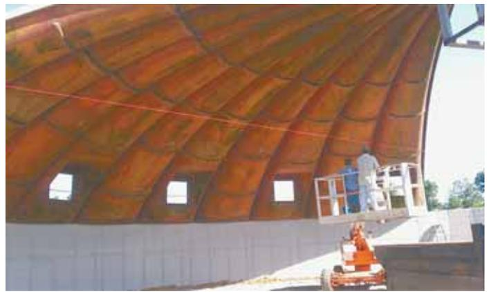
They hired a crew with a 100-ft. boom to set the 50-ft. long panels on 10-ft. high, 1-ft. thick concrete walls. Every other panel has a 3-ft. sq. opening for ventilation.
