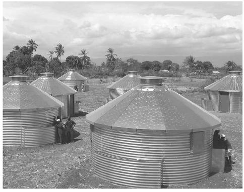
they can easily be transported by hand or on carts. They include two windows and a door. The lip at the edge of the first layer of the 24-gauge steel roof is turned up to help channel water for collection under the eave. The top heat shield layer is made of perforated steel that shades the roof. The double roof combined with a cupola and continuous ventilation under the eave, keeps the unit cooler than outside.
