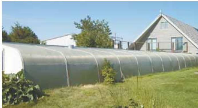
“Underground” greenhouse is buried 5 ft. below ground and measures 80 ft. long by 16 ft. wide. It uses earth heat as the only source of heating and cooling.
