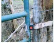
Seat belt is lag screwed to gate post. Pulling on the strap snugs the gate up tight.
