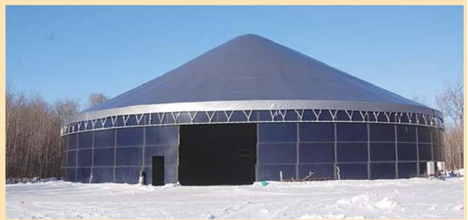
Project manager Paul Hofer reduced the slurry tank's 23-ft. high walls to 18 ft. and cut out holes for an entrance door and overhead door.
