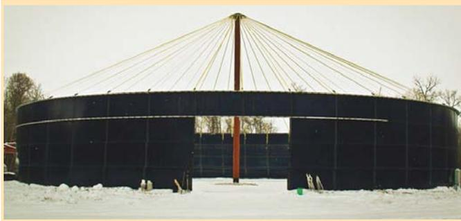
A Hutterite Colony in Manitoba used ratchet straps and custom-sewn canvas to enclose this former 120-ft. dia. slurry tank.
