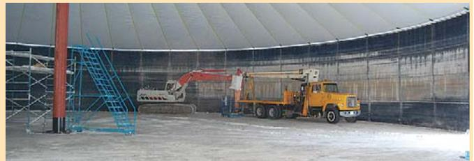
Inside, he installed a 50-ft. tall, 20-in. oilfield pipe at the center. A 5-ft. dia. steel frame is welded onto top of pipe.
