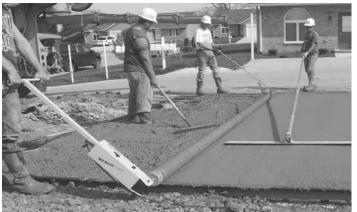
Spin Screed engineers have developed a "Gutter Builder" screed that can be used to build drive over curb and gutters and valley pans in a single pass.
