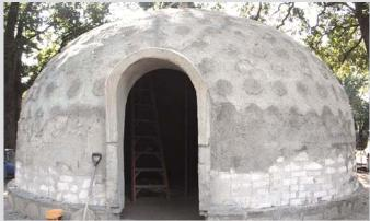
Dome building system uses a lightweight cement mixture with poly beads and an inflated "balloon" form. Air-filled beads reduce mixture's weight and improves insulation.
