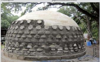
Dome is shown here partially completed with scaffold and air form inflated.
