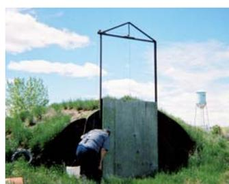
Plywood door raises straight up and down a tall metal frame, and is lifted by a shop drill attached to an electric winch.
