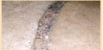
Cracks in asphalt driveways and concrete floors can be filled with expandable spray insulating foam topped with crack filler and grit, says Roger Meihak
