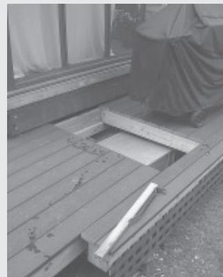
Second Rain water "barrels" are designed to be concealed under patio seating in plant stands or under decks.
