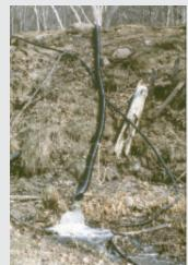
Water swooshed out lower end of pipe. plug right through the pipe and out the other end as well. The siphon quickly lowered the water to a safe level.
