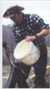
To keep his farm pond from overflowing, Art Briggs-Jude used a 50-ft. section of flexible 4-in. drain pipe as a giant siphon. He sealed off the bottom, left, and filled the pipe from the top using a 5-gal. bucket.
