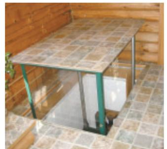
Top of elevator is finished off with floor tiles that match the floor above.
