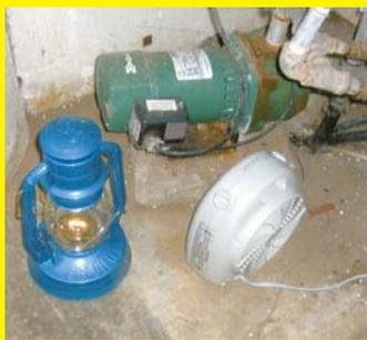
I keep an oil-filled Dietz lantern around the farm for emergency heat. For example, a lantern will keep my small insulated pump house warm for up to 30 hours on one fill. As a bonus, you can use the lantern for light any time of the year that the power goes out. I bought the lantern shown here on the internet for about \$40. **(C.F. Marley, Nokomis, Ill.)**
