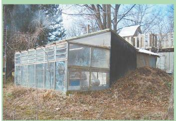
Greenhouse is built into side of hill, with heat from the ground keeping the greenhouse warm. Accment mixer drum is buried in the hill side behind it.
