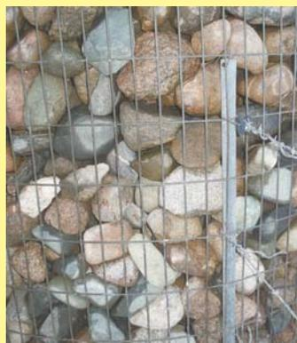
He uses wire panels from old corn cribs to make the cages, wiring the panels to metal posts.
