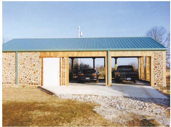
Greg Van Winkle built this garage using cordwood and a concrete mix that included sawdust.
