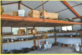
Kenny Cemper builds lowcost sheds out of discarded irrigation pipes.
