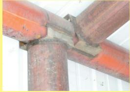
He joins vertical and horizontal pipes together with angle iron brackets.
