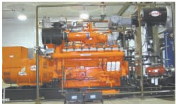
Heat recovery unit, right, produces hot water using “waste heat” off this stationary diesel-powered generator.
