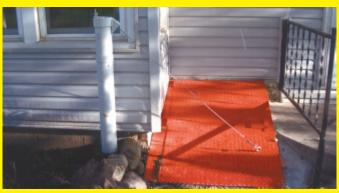
By making use of a counterweight I was able to come up with an easy-open "pit door" for the outside entrance to the basement at our daughter's place. The door is made from 1/8-in. thick deck plate and was too heavy for her to lift. I didn't want lag screws, pulleys, etc. screwed into the house, so I built a counterweight system as shown. It takes all the work out of lifting the door.
