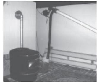
Joseph Rupinski built a large corn bin (left) in his basement that supplies his corn burning stove via an electric feed conveyor (right). Screw conveyor runs from bin to flexible plastic filler tube.
