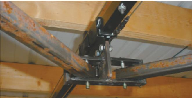
Metal bracket is attached to opener's chain and rides back and forth along the rail.
