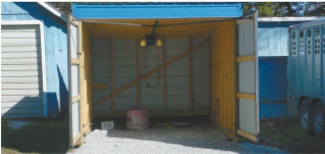
Glen Schewpe uses a single garage door opener to open a set of double doors on his home-built garage.
