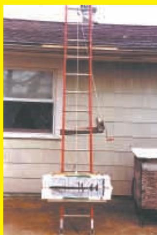
Hauling 50-lb. packs of roofing shingles up a ladder can be hard work. To make the job easier I use a hand-operated winch attached to a board on back of the ladder. Cable from the winch leads up to a pulley on the ladder's top rung, and then back down to an L-shaped wooden carrier with a hook on top of it. Four small metal trolleys on back of the carrier keep it from accidentally sliding off the side of the ladder.
