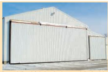
Door opens in 35 seconds. Lock valves and restrictors prevent the doors from closing
