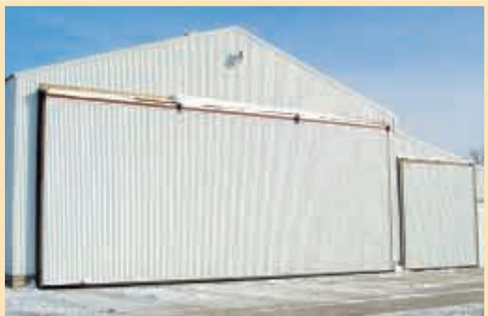
Door opens in 35 seconds. Lock valves and restrictors prevent the doors from closing in less than 30 seconds, even if system fails.
