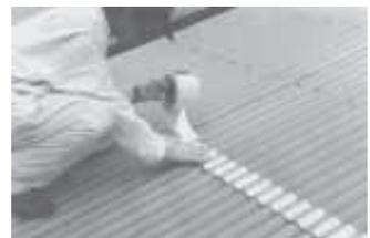
Peel & Seal roofing is an aluminum-backed, rubberized asphalt product that you simply roll out and stick in place.
