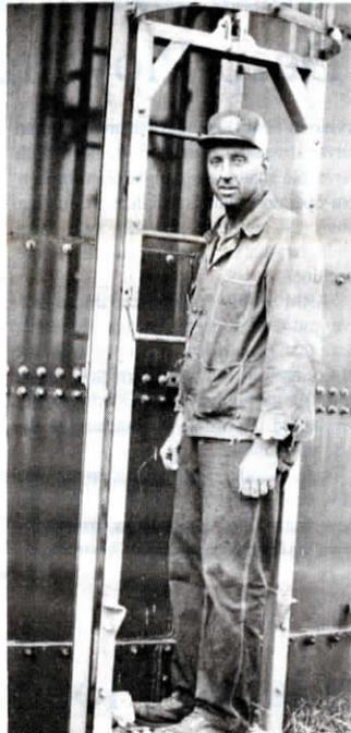
Note counter-weight (top) which offsets Roger Schnell's weight, plus the weight of the carriage.
