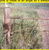
comes back to center. It opens when bumped by a vehicle and automatically swings shut after the vehicle passes through. An insulated tip allows the gate to be opened by hand.
