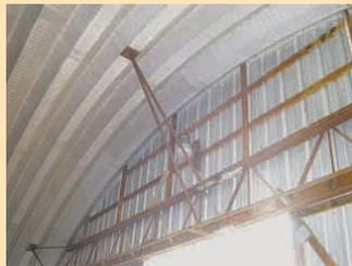
Ickes got a used roof truss out of another large building and turned it upside down. Because the upside-down truss is top heavy, he ran a brace to each corner of the building and also in the middle.
