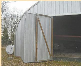
Tri-fold doors slide on a pair of conventional barn tracks, with each track covering two doors. The two inside doors are hinged and swing out.
