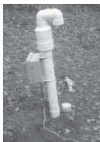
**Septic Heater simply slips onto vent pipe above tank or drainfield. Control box turns heater on and off as needed to keep system from freezing.**
