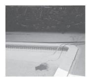
A submerged pump circulates water through the solar heated hose.
