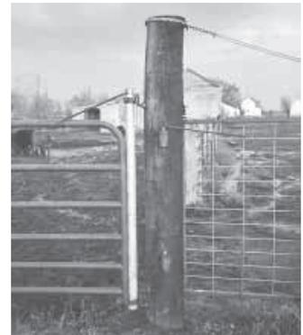
Post welded to gate is 2 in. below and 1 ft. above it, which puts the hinge bolts further apart. This stops gate from sagging.
