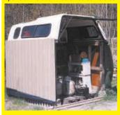
to the outside of the skids and added some caulking to make the shelter water-tight. By setting the walls on a 2 by 6 bottom plate, I can use a truck or tractor to tow the building to a new location. (Louis Trepanier, Rt. 2, Haliburton, Ontario. Canada KOM 150)
