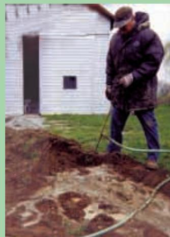
**Lyle Dawson's "soil compactor" is a 4-ft. long hollow metal tube that hooks up to a garden hose. Water exiting from the end of pipe saturates the soil, penetrating to bottom of trench.**
